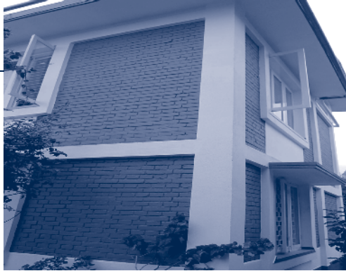
Existing building retrofitted with external beams and columns
