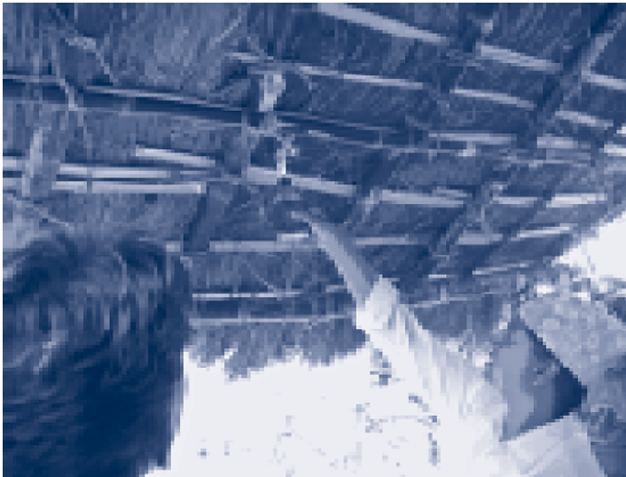
Testing fire resistant thatch roof
