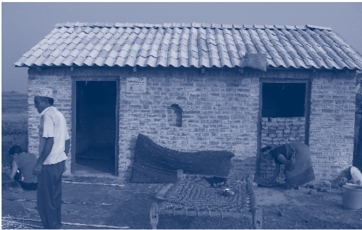
House constructed by Caritas for fire victims in Butwal
