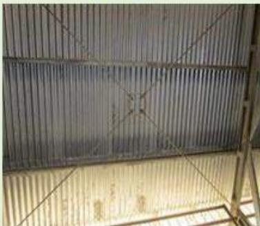
Steel bracing to roof
