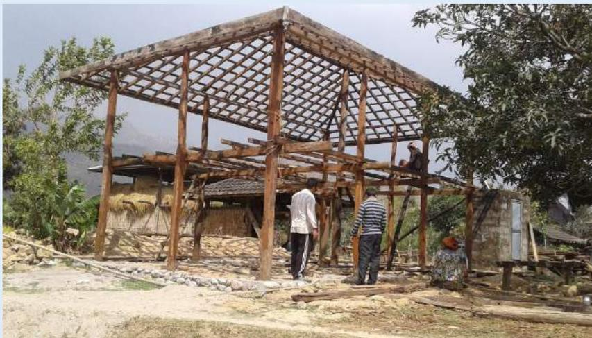
Wood is light construction material with high strength, therefore, is highly preferred material in construction. However, heavy cladding walls increases loading demand laterally on a frame beyond its structural capacity.
