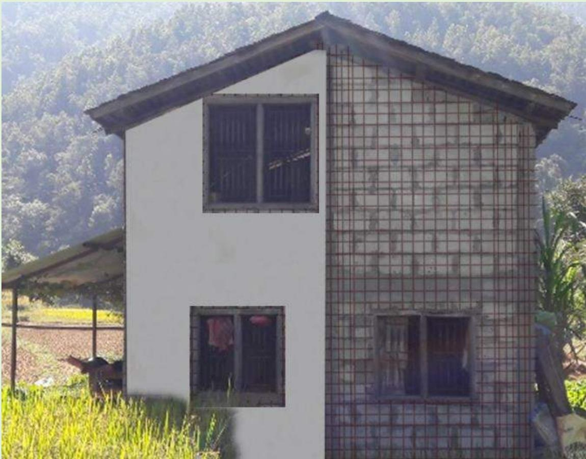
Figures : Jacketing of HCB building using GI wires and plaster
