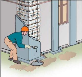
An illustration showing a construction worker in a blue shirt and orange hard hat applying micro-concrete to a wall. The worker is using a hand tool to spread the material. The wall has a grid of reinforcement visible. The floor is covered with a protective layer. |
