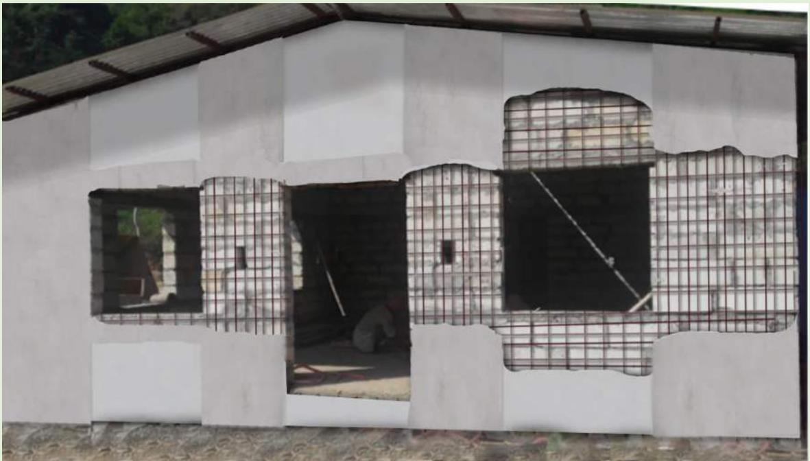
Figures : Jacketing of HCB building using GI wires and plaster
