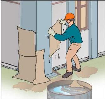
An illustration showing a construction worker in a blue shirt and orange hard hat applying jute bags to a wall. The worker is standing next to a bucket of water. The wall has a grid of reinforcement visible. The floor is covered with a protective layer.           |
