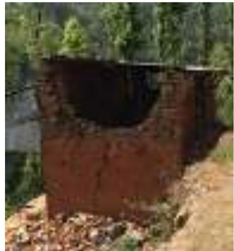
Damage of stone masonry gable wall
