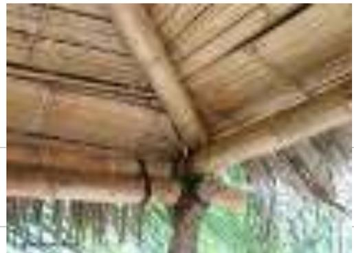
Vertical, Horizontal & Diagonal members connection using Lacing (Jute, Lylon, or equivalent) Techniques
