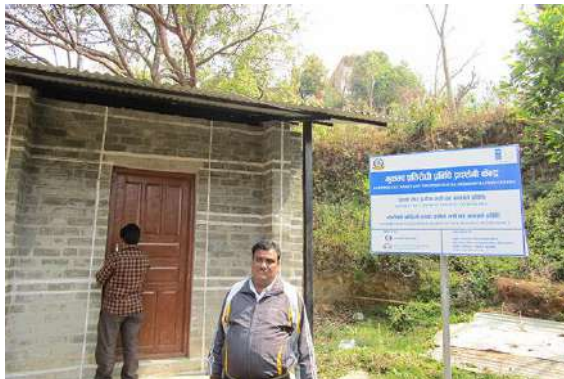
Compressed Stabilized Earthen Block (CSEB) Demonstration House, Saraswati HS School, Gorkha Bazaar, Gorkha
