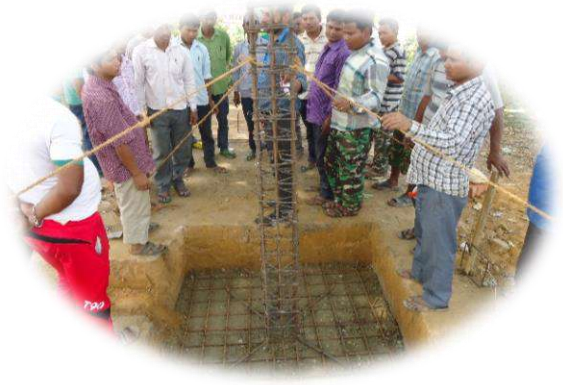
Masons in practical session of safer construction training, Maadi, Chitwan
