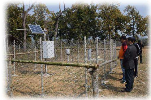
Figure 2 EWS Station, Riu-khola, Chitwan
