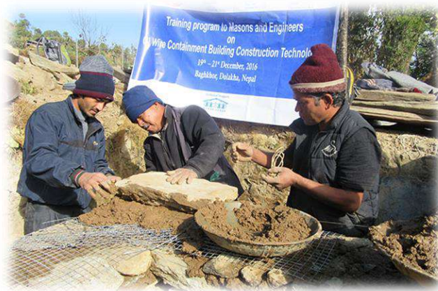
Trainees of GI Wire Containment training, Katakuti, Dolakha
