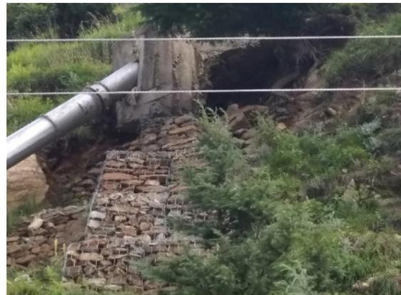
*Figure 11: Gabion wall for the maintenance of local electricity powerhouse in Jumla*
