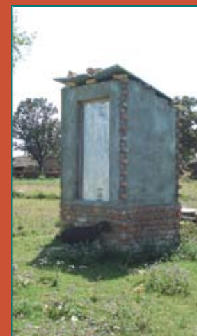
High Plinth Level of Latrin for Flood response, Rupandehi. Photo: Eco-Nepal
