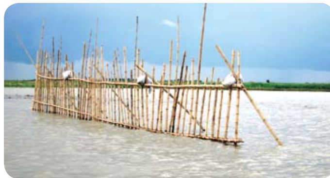
Bamboo binding is an efficient adaptation strategy used by the farmers of Sonatoni. They are building bamboo fences, or Chatka , to redirect the river to prevent soil erosion. This way they have gained about 400 acres of land in only two years. Photo: Anette Wilhelmsen/LI-BIRD
