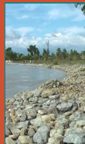
River channeling. Gabion wall Koshi flood Photo: Eco-Nepal
