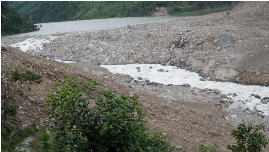
The landslide-Dam and the part of the lower end of the lake . Viewed from the downstream side. (photo: Hari Darshan Shrestha)
